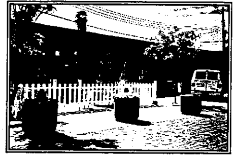
Municipal Parking- Rear Building Facades
