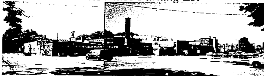
Existing rear parking lot at Curtiss Place
