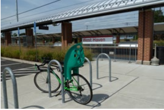
West Haven Station
